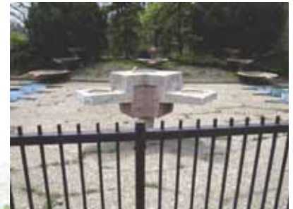
Lott Memorial Fountain Project - existing Photo credit: Lisa Kemp
